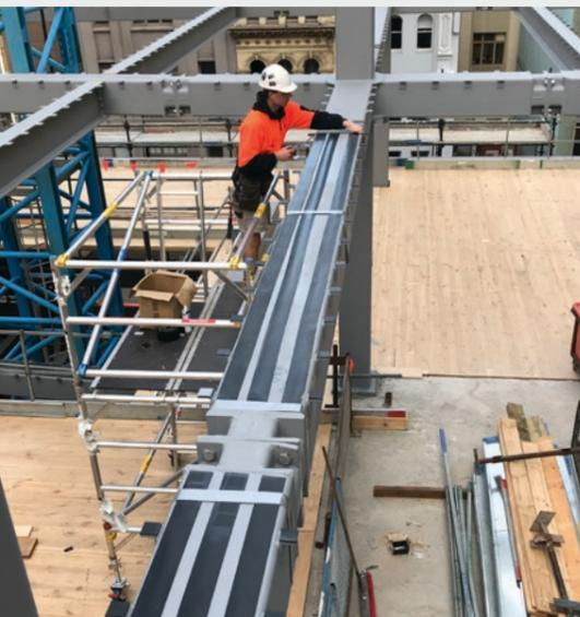
Positioning of neoprene 60 HG rubber strips on steel beam joists.
